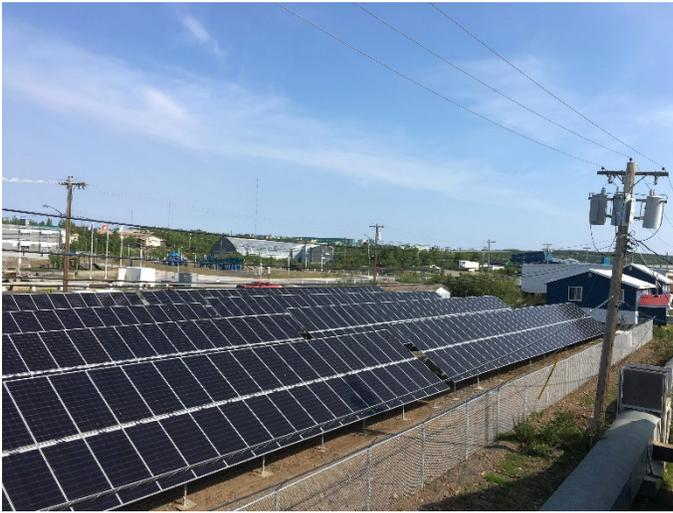
In 2018, Solvest worked with the Nihtat Gwich'in Development Corporation to install various PV systems in Inuvik, NWT. Solvest designed and installed 32 residential Gwitchin owned houses as well as two commercial PV systems. These commercial systems are “behind the meter”, meaning production was matched up with base load using smart controllers, to ensure no export to the grid.
