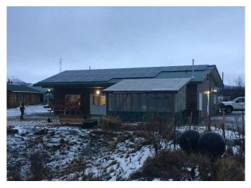
In 2019, Solvest installed a 23kW solar array along with a 90kWh battery bank, designed to power the Kluane Lake Research Station (KLRS). As this location is remote, battery was specifically designed to be able to freeze to -68°.
