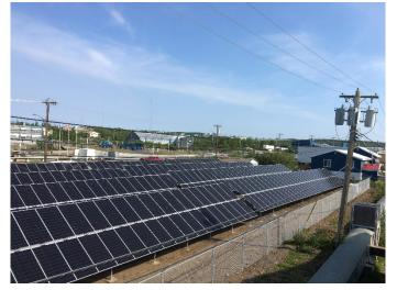
In 2018, Solvest worked with the Nihtat Gwich'in Development Corporation to install various PV systems in Inuvik, NWT. Solvest designed and installed 32 residential Gwitchin owned houses as well as two commercial PV systems. These commercial systems are "behind the meter", meaning production was matched up with base load using smart controllers, to ensure no export to the grid.
