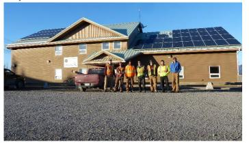
In March 2016, Solvest was selected to construct roof top solar arrays totaling 43kW for Kluane First Nation. Due to budgetary year end requirements, this project had extremely tight timelines requiring the arrays to be designed and installed within 30 days. Solvest designed three solar arrays for adjacent Kluane First Nation buildings, two 15kW installations, and one 13kW installation.
